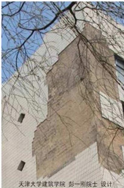
**Figure 8** Ceramic tiles falling
